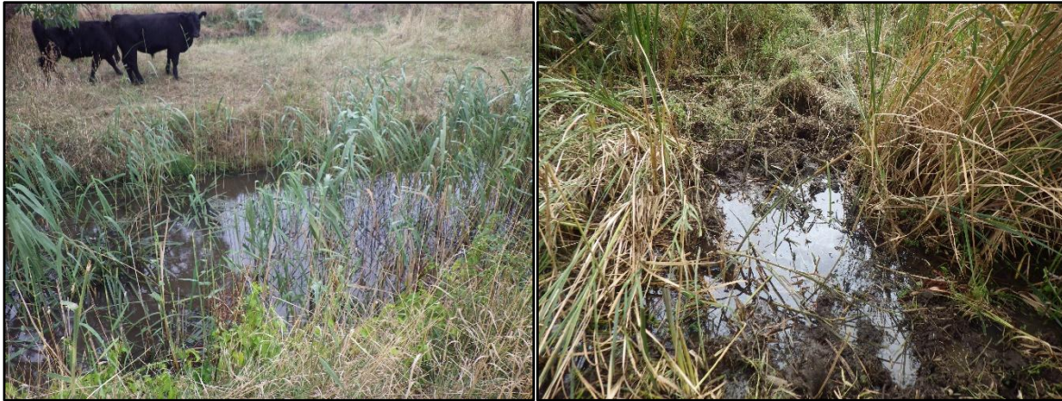
Figure 10. a) Stock access and b) associated damage in the lower Finniss River (Winery Rd) in autumn 2014.
